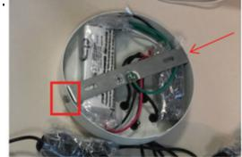
2. Depending on the length needed to run FLAP LED power wires behind wall, cut wires at appropriate length (approx. 7" from housing); strip plastic to expose copper wire ends
